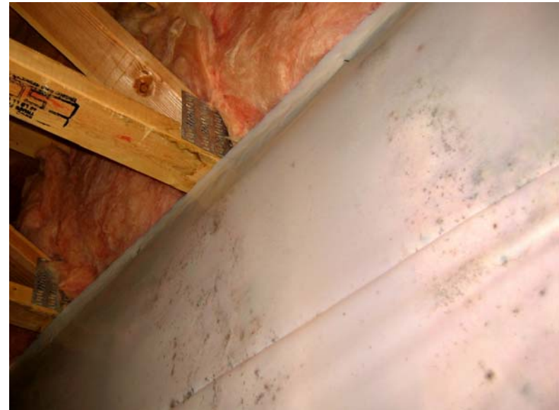
Photo - Rear wall plastic sheeting
